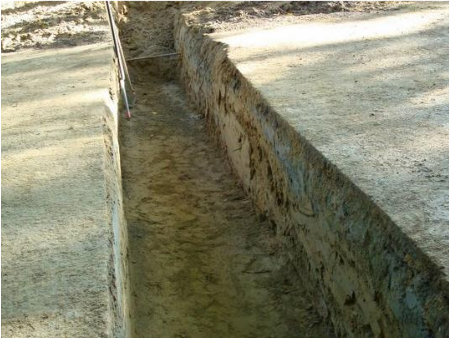
Culvert trench under 38 th . Notice how sandy the soil is here.
