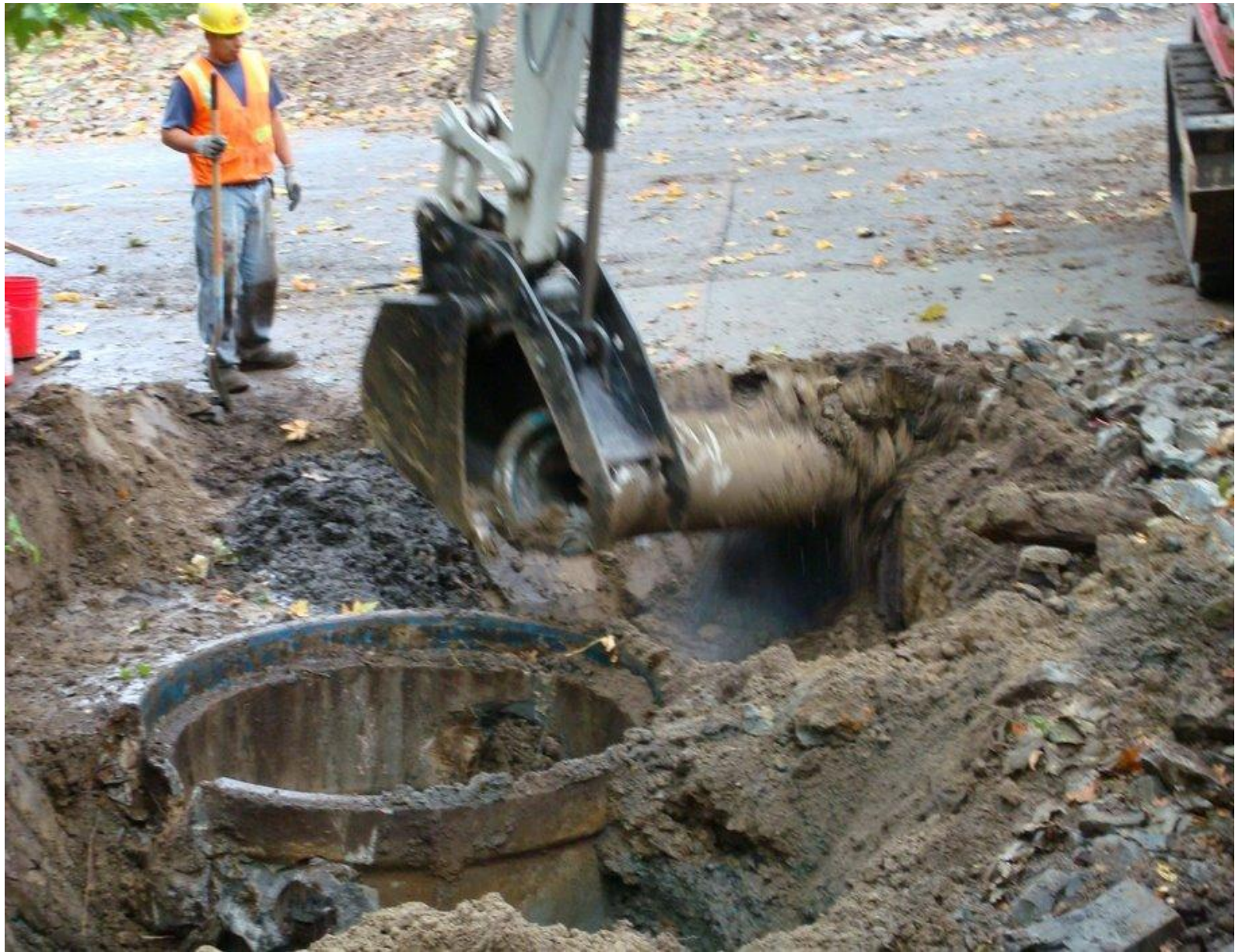
Removing catch basin above 38th
